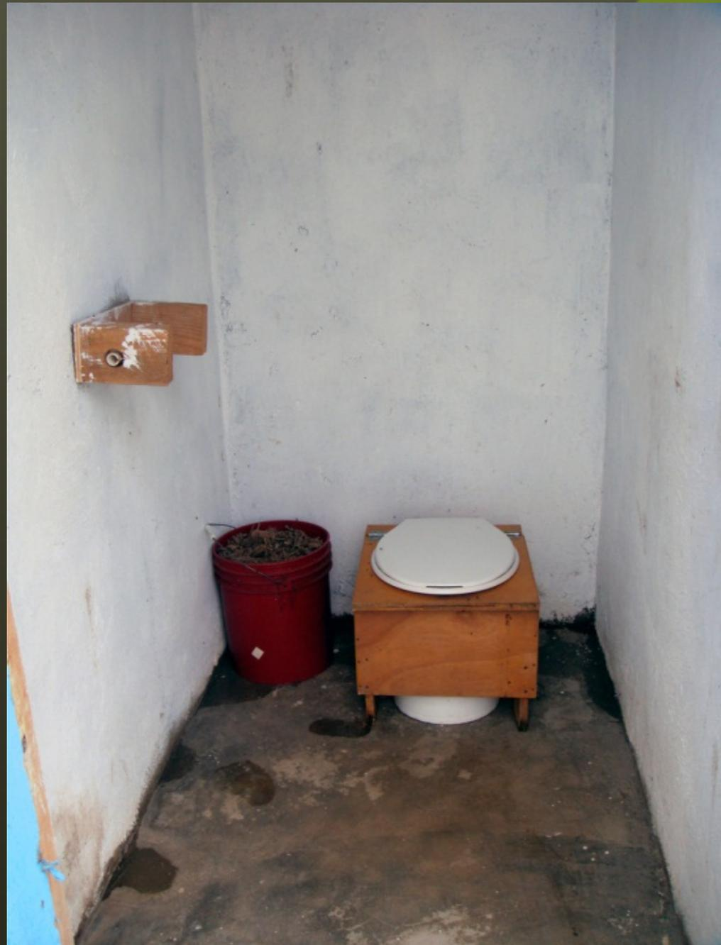
The contents are covered with a carbon-based material. The receptacle is easily removable.
