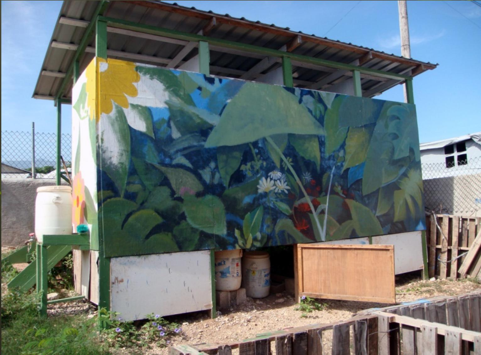
One drum is being filled while an empty one waits to replace it.
